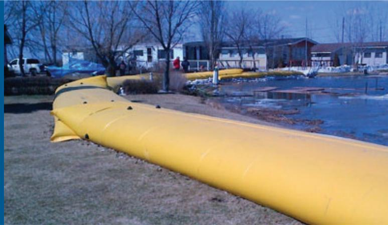
***Nilex's water inflated dam provides a rapidly deployed, temporary flood solution.***
