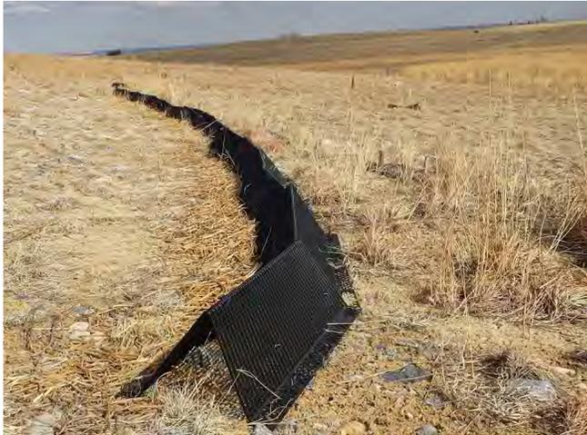
The client purchased 1,340 sections of GeoRidge, and the contractor has been installing it with crews of two, using 10-inch landscaping spikes. It was installed in drainage channels to slow water velocity and limit erosion as well as along the contours of slopes to control sheet erosion, which is generally harder to control because it can take longer to recognize.
