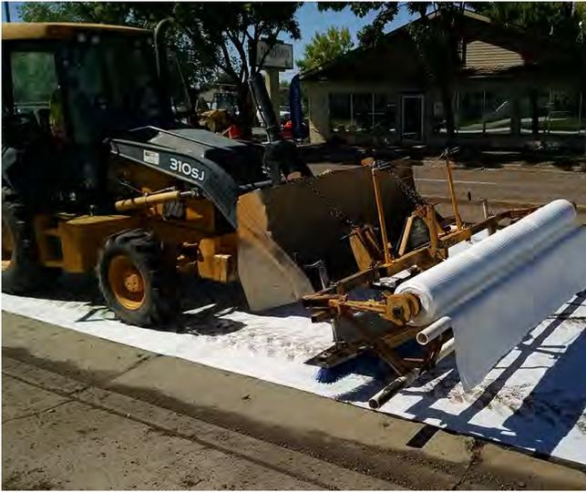
Rainy and cold conditions required a change in tack coating to ensure the mats adhered to the road surface, otherwise, applying the mats proved to be one of the smoothest parts of the project. Nilex was on site to assist with this work. Four people were involved in the mat installation, ultimately using 69,000 square yards (approximately 58,000 m<sup>2</sup>).
