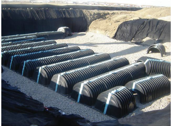
There was significant savings on this project using Nilex's recommended stormwater management system. Installing the chambers underground capitalized on space, allowed for greater runoff storage and, maximized the number of parking stalls on the property.
