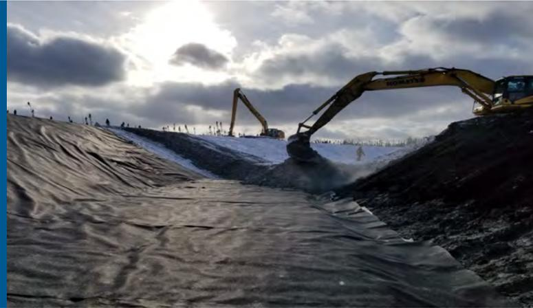
**Geosynthetic Clay Liners (GCL's) are high performance environmental liners used in environmental containment applications. One truck load of GCL's is equivalent to 150 truckloads of compacted clay.**
