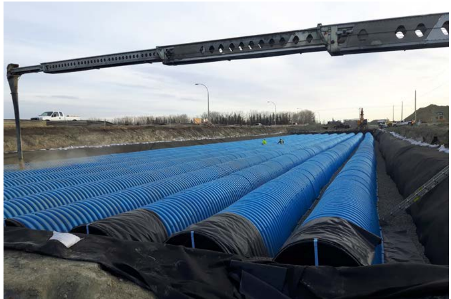
Underground stormwater detention systems can eliminate the need for on-site stormwater ponds.
